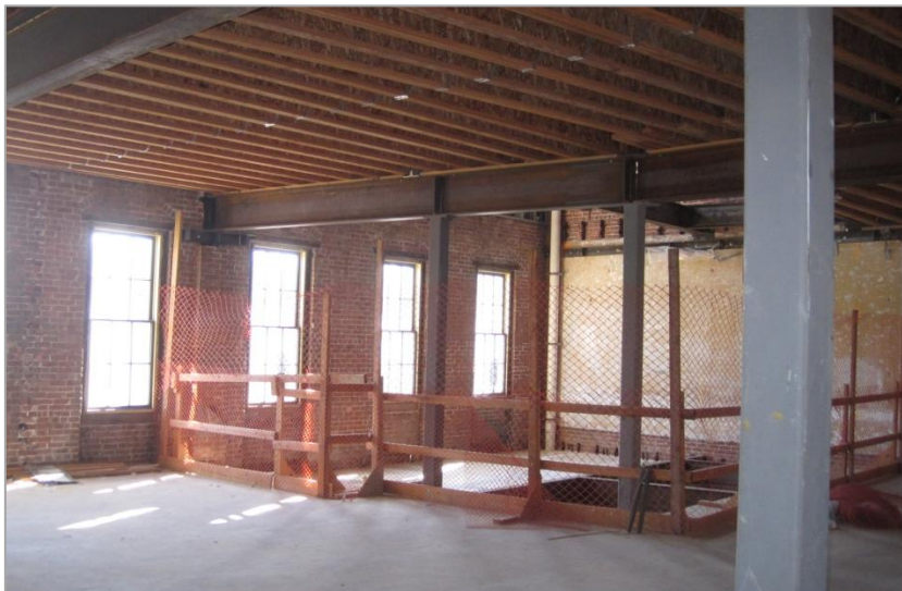
Existing Opening (Elevator Shaft)
