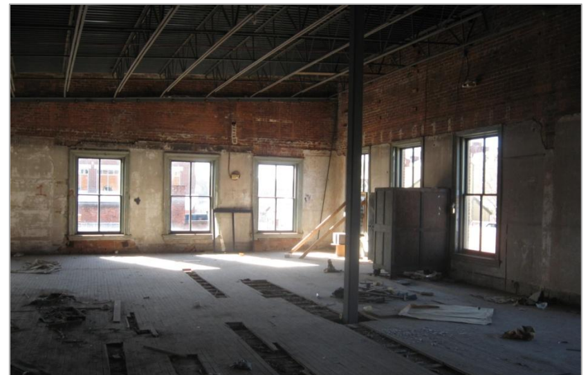
Interior of an Upper Floor
