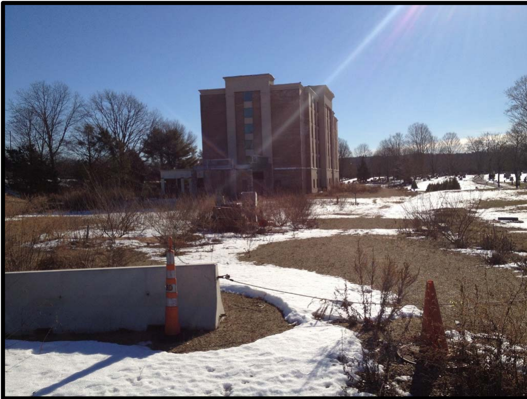
North elevation incomplete site work incomplete
