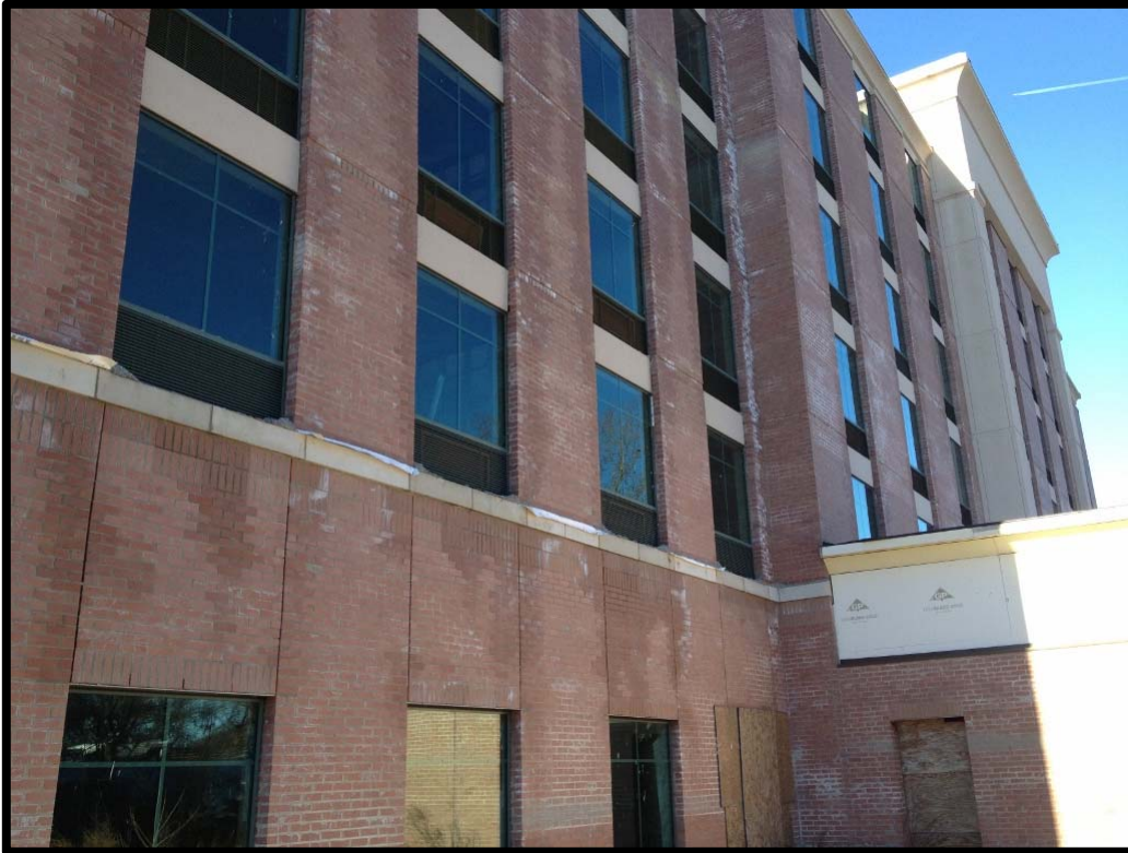
East elevation at the south end of the building facing Interstate 395
