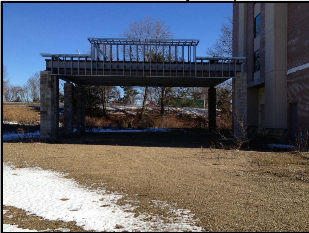
Canopy at north elevation incomplete
