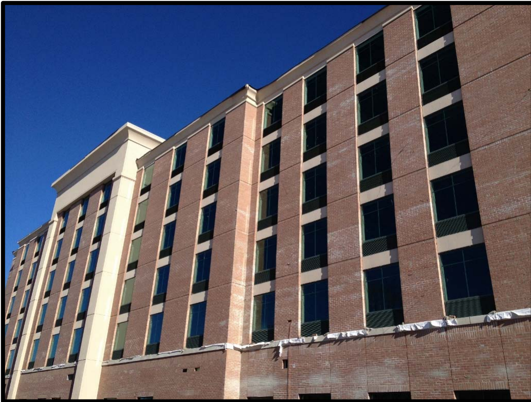
South elevation overlooking a cemetery
