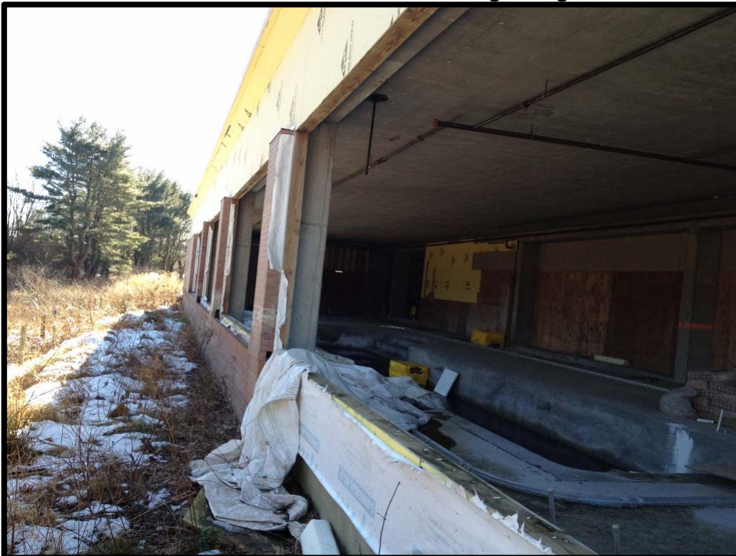
Unfinished exterior and pool room along the east elevation
